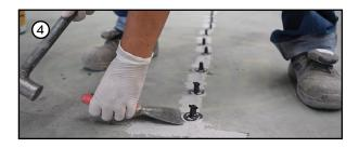
4) Remove the plate after injection epoxy is finish 2-3 hours.
