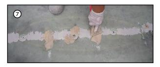
7) Putty closed Ferrostud 6 mm. with waterbased epoxy adhesive (Ferrorez 711) let dry 6 hours.
