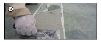
9) Plastering decorative cracks to be smooth with decorative mortar (Ferropatch 551) let dry 1-2 hours. In case on is not pour top layer with Ferrocrete 216.
