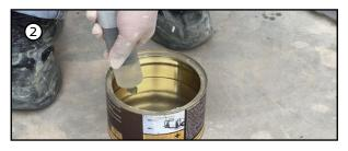
2) Fill the resin mixture into cylinder injector within 3-5 minutes after mixing.
