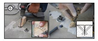
6) Holes with a drill use an oblique guide of 55-60 degrees. to form a cross. Away from the crack 1 inch, depth 15 cm. Mixing water -based epoxy adhesive (Ferrorez 711) on steel and inlaid Deformed bar SD40 DB 12 mm. \*13 cm. space 50 cm.
