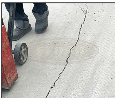
Concrete cracks before injection repair.
