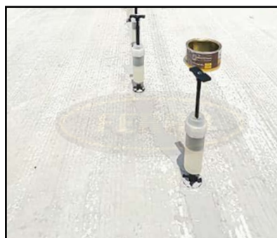
Injection cracks repair with super fast acrylic crack repair (Ferrorez 700/KIT) or crack injection kit for concrete repair (Ferrorez 717/KIT).
