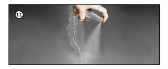
11) Leave to dry, curing spray with clean water or Ferocure 105 Lithium silicate.
