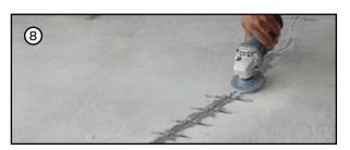
8) Grinding the crack line to make a uniform to the concrete surface.
