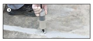
3) Twist the axis of the cylinder a little and pushing the resin in the cylinder down to the plate. Then slowly seeped into the cracks wait 20 minutes when see that the injection is not down, remove and wipe with xylene and can be injected again 1-2 times.
