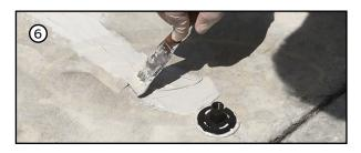
6) Stick follow along the cracks and edges with Ferrorez 717/GL/600 g. Fast-Setting glue for injection plate (Size 600 g./set) leave dry 2-3 hours.
