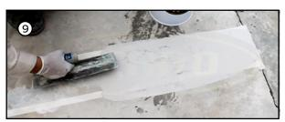
Plastered decorative cracks to be smooth with crack repair mortar Ferropatch 551 Decorative mortar.
