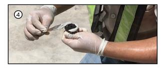
4) Plastered Ferrorez 717/GL/600 g. Fast-Setting glue for injection plate (Size 600 g./set) under plasterd Ferrorez 717/CP/50 ml. (Cylinder 50 ml. & plate).
