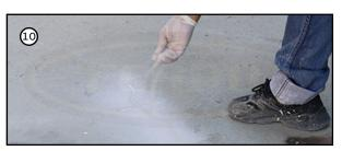
10) In case original concrete surface has color can be sprinkled with colored powder iron oxide type such as green, red little while Ferropatch 551 Decorative mortar began to dry. If you want the colour similar to the colour of concrete adjacent. Beware careful of splitting the sesame crack if you sprinkle too much colour powder.
