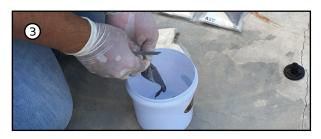
3) Use Ferrorez 717/GL/600 g. Fast-Setting glue for injection plate (Size 600 g./set) mixing ratio A: B1:1 fast-setting 2-3 hours.
