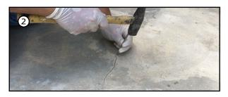
Calculate the distance to place the plates (Estimate distance 20-30 cm.) and open drop point Ferrorez 717/CP/50 ml. (Cylinder 50 ml. & plate) open crack surface at the plate point by chiseling.
