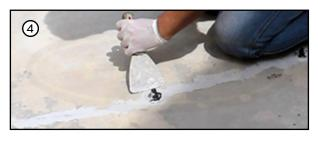
4) Remove the plate after injection epoxy is finished 2-3 hours and cover the plate with Ferrorez 717/GL/600 g. Fast-Setting glue for injection plate (Size 600 g./set) and leave dry for 2-3 hours.
