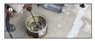
1) Mixing part A: 1.6 kg. (1600 g.) and part B: 0.4 kg. (400 g.) mixing with low speed driller 1-2 minutes until homogeneous.
