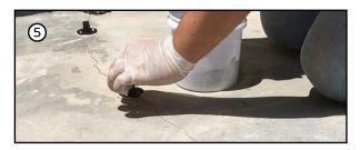
5) Install Ferrorez 717/CP/50 ml. Cylinder 50 ml. & plate) over the opened point.
